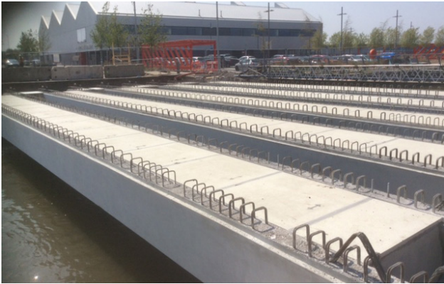
Bridge Construction at Birkenhead for the re development of Liverpool Docks
